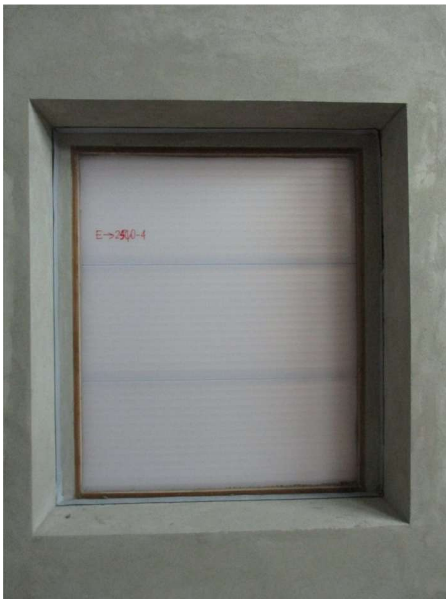
Photograph of item, receiving room side
